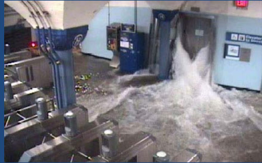
PATH – Hoboken Train Station
